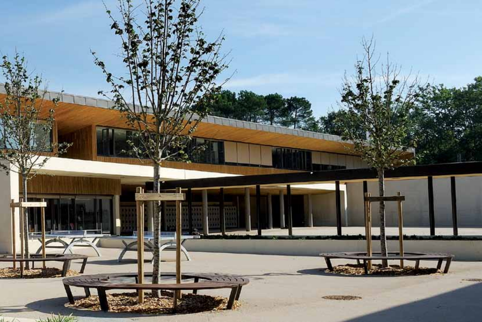
Saint-Paul-lès-Dax College - Architect: Cabinet Hubert Photography: P. Loubet
